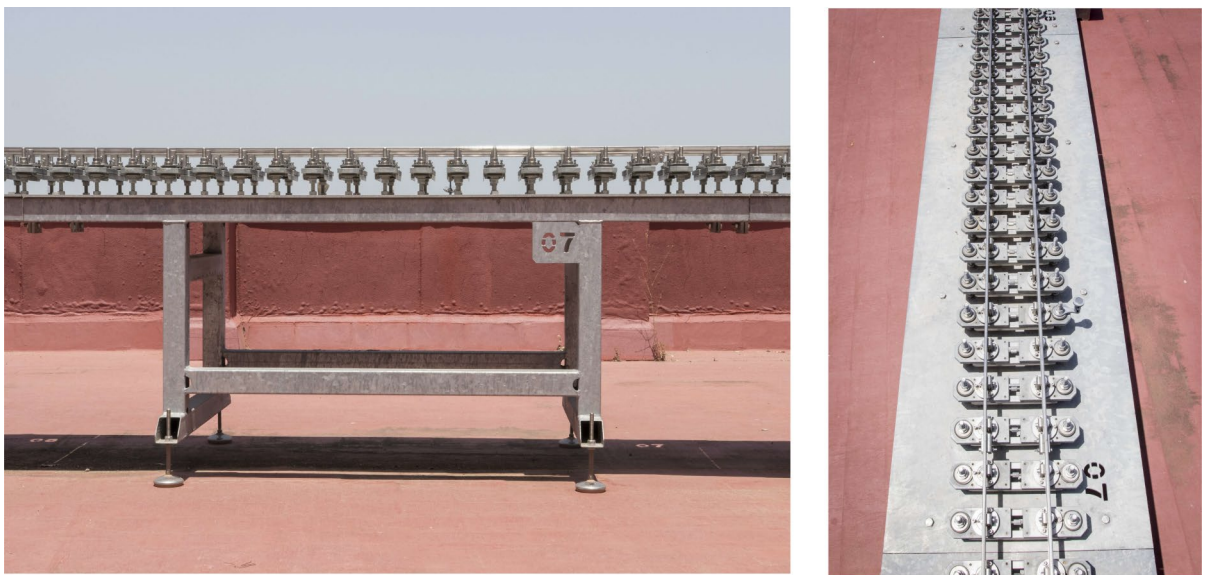
Figure 9. Table support structure: elevation view (left); horizontal view (right). Photographer: Ludivine Mimar.
